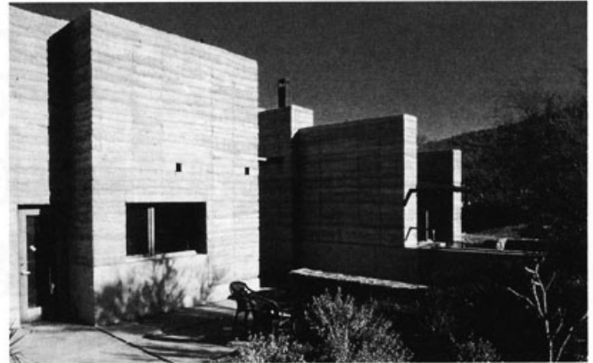
Exposed cement-stabilized rammed earth form the 24-inch-thick (610 mm) walls of this house in Tucson, Arizona.
