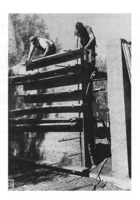
Forms are being removed from a section of 16-inch-thick (406 mm) rammed earth wall, just completed in central New Mexico. In this case, extra thick sheets of oversized plywood serve as forms, with whalers of 2-inch by 10-inch (51 mm by 254 mm) lumber, and pipe clamps to tighten the assembly. These walls become hard enough to bend a No. 16 nail within two days of exposure to the air.
