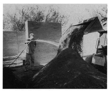
A New Mexico crewman uses a spray attachment to water down a pile of prepared soil, as it is turned by the Bobcat. Prior to adding the water, the dirt is dry-mixed with a premeasured amount of portland cement. The pile represents the amount of work that must be done (rammed) within 90 minutes of mixing. The objective is to bring the mix to roughly a 10 percent moisture content, with a uniform color and texture.
