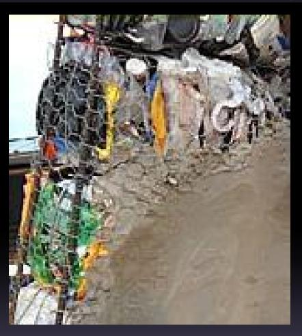
Use plastic fishnet or galvanized chicken wire tied to rebar
